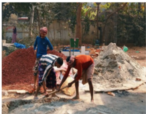
Picture above shows the washroom construction has started on the temple site inside Jagannath University.
