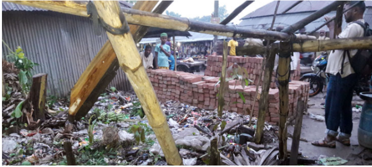
Samir Bhakta's tea shop in Pakhimara Bazar, Narail destroyed
